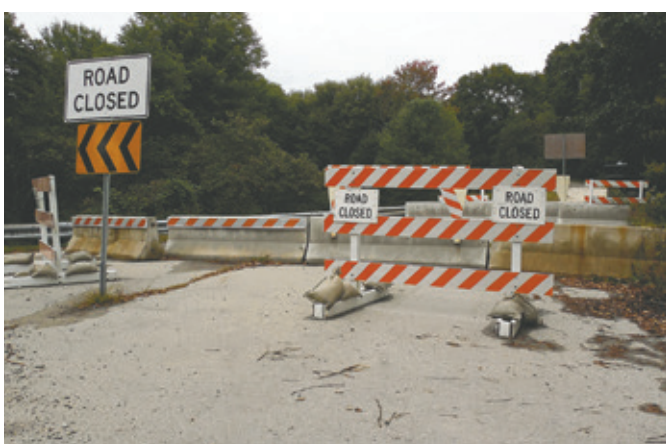
Barricades and detour signs remain in place... for now
