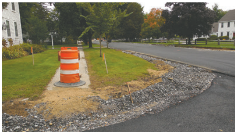
Progress: Corner of Boston Post Road and Cross Street, Amherst Village
