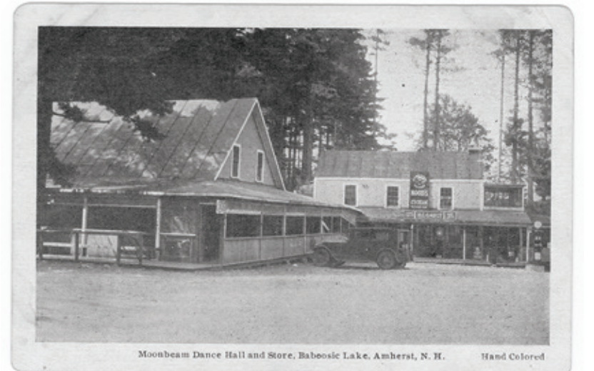
Moonbeam Dance Hall and Store, Baboosic Lake, Amherst, N. H. Hand Colored Moonbeam dance hall at Baboosic Lake, c. 1935. Originally built 1903 by Louis E. Clark, it was rebuilt in 1931, after collapse of snow-laden roof, by Harold C. Gault, who owned Moonbeam and store next door 1926 to 1936.
