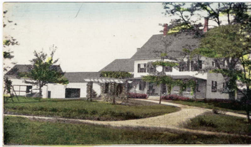
Published by G. F. Wenzel & Son Point of Pines House, Baboosic Lake, Amherst, N. H. Point of Pines hotel overlooking Baboosic Lake, Amherst, N.H., built in 1873 with four rooms downstairs and 12 sleeping rooms above; burned in 1939. Photo after 1914; postcard published c. 1930.
